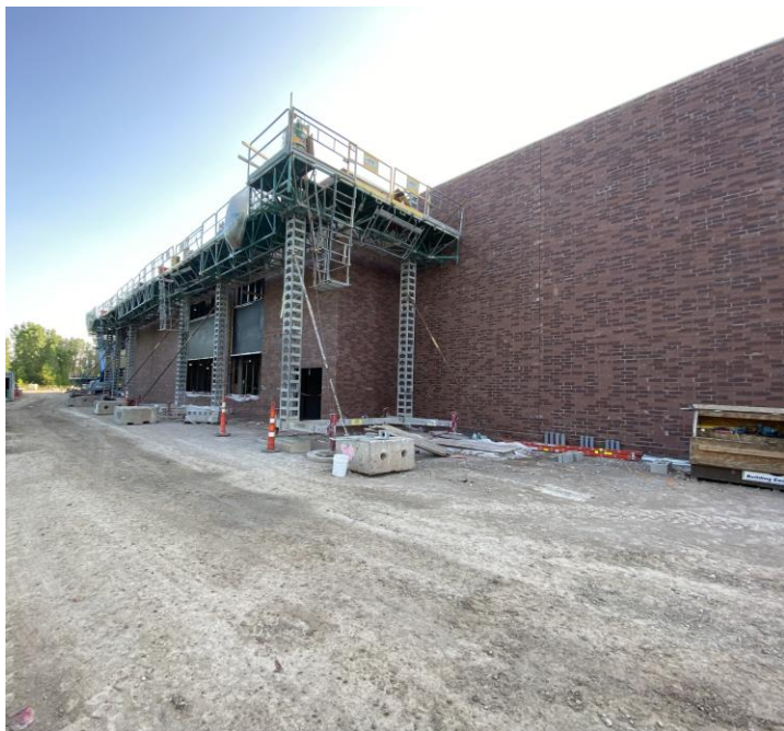
Exterior brickwork is nearing completion on the building's west side.
