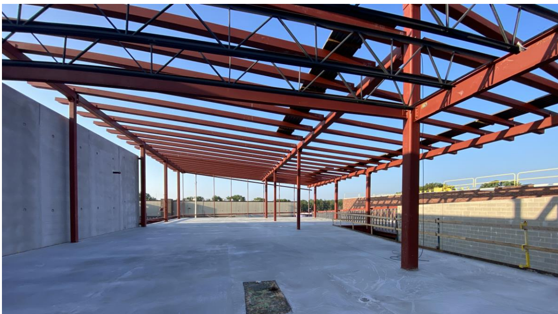
The structural steel framing of the library is in place and the floor has been poured.
